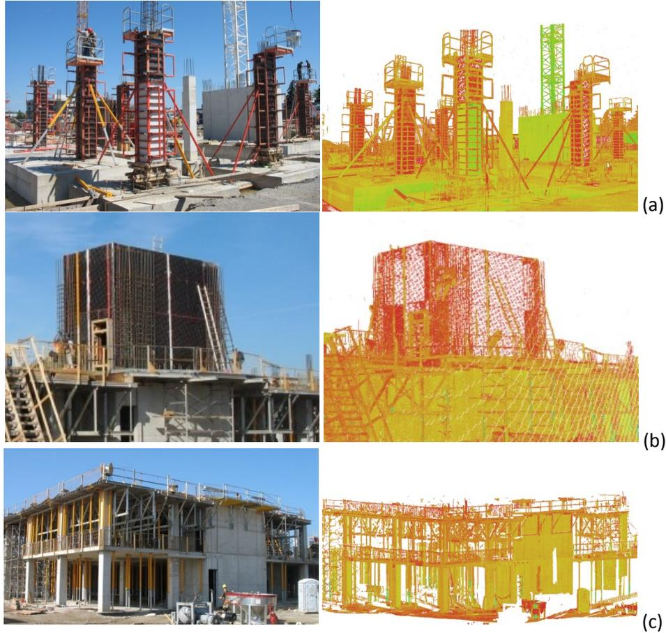
**Figure 3: Temporary and Secondary objects at E5 Building site: (a) column formworks – July 25, 2008; (b) Rebar – September 19, 2008; (c) Slab formworks and shoring – October 9, 2008.**
