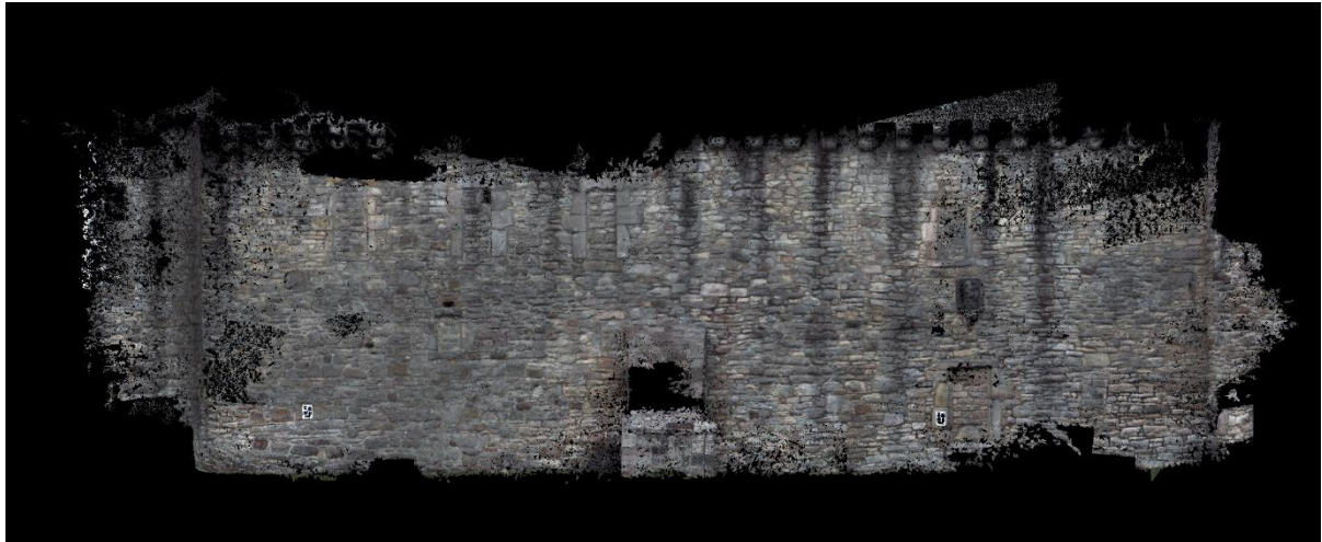
Figure 21: Point cloud of the rampart wall facing the East garden obtained by the pole-mounted stereo system.
