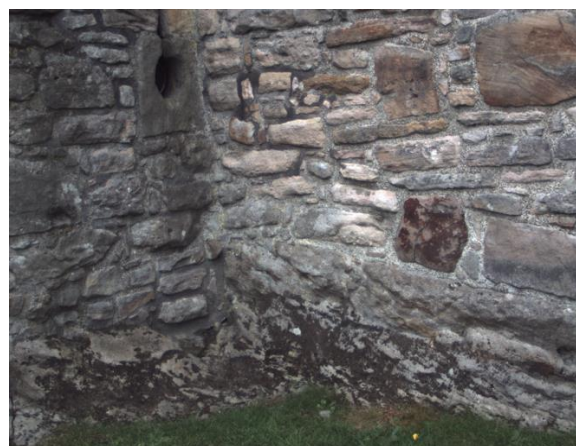
Figure 33: Area between the main wall and a tower.
