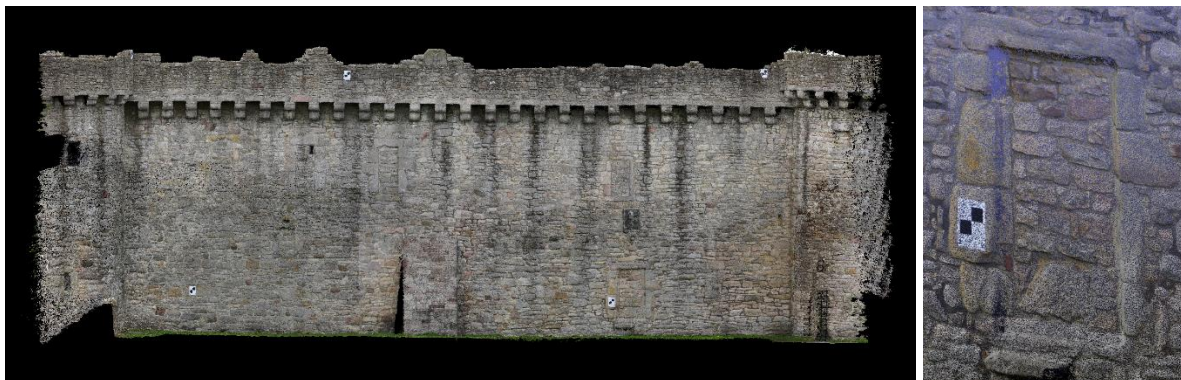
Figure 19: Main wall of the East garden obtained by the Sony camera. Right: detail of a window.
