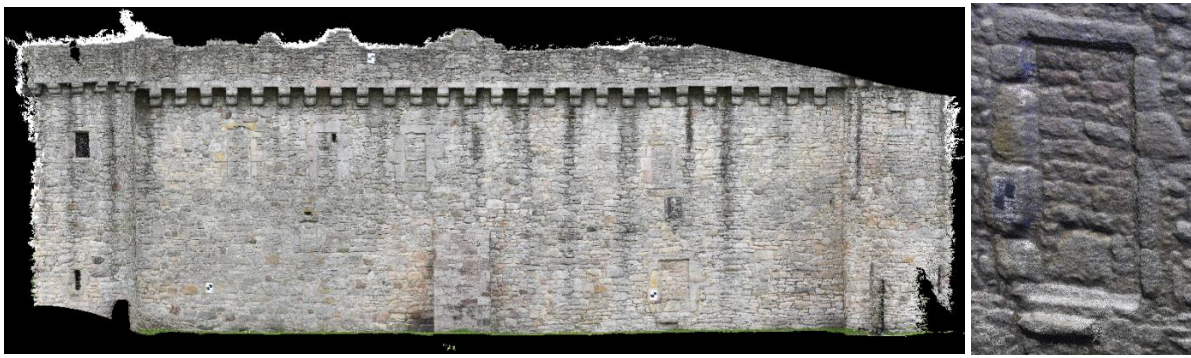
Figure 17: Point cloud of the rampart wall facing the East garden obtained by the pole-mounted Nikon camera. Right: detail of a blocked-up window. The point cloud is coloured with the true colour acquired by the camera.
