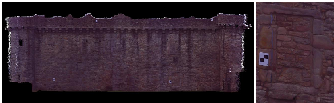
Figure 15: Point cloud of the rampart wall facing the East garden obtained by the Faro Focus 3D TLS. Right: detail of a blocked-up window. The point cloud is coloured with the true colour acquired by the scanner.
